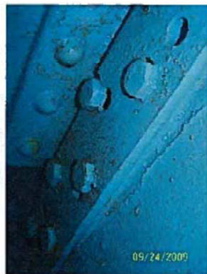
Typical view of previously rehabed diagonals. Having problems were the bolt holes had to be redrilled during the rehab.
