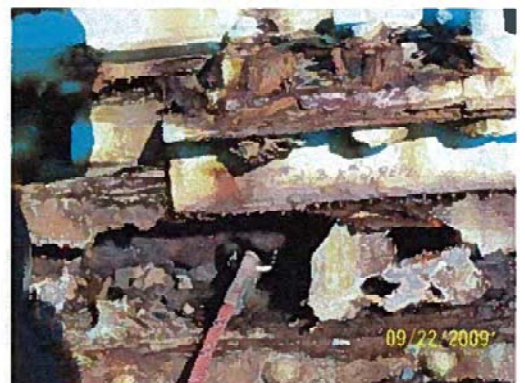
Exterior view of bearing device #2 at Pier #2. Bearing device needs to be replaced.
