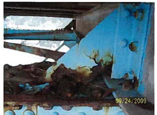
Typical view of floor beam bracing. Most have heavy section loss and some braces are completely gone or broken.
